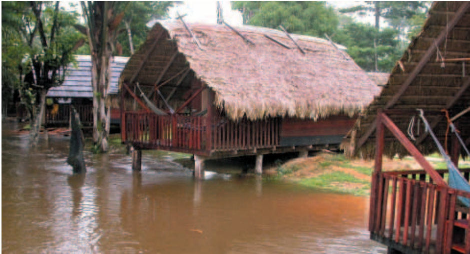
Severe flooding in 2006
