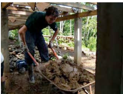
Expanding the technical college facilities
