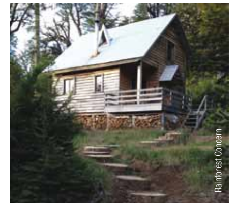
Newly completed cabin for research students
