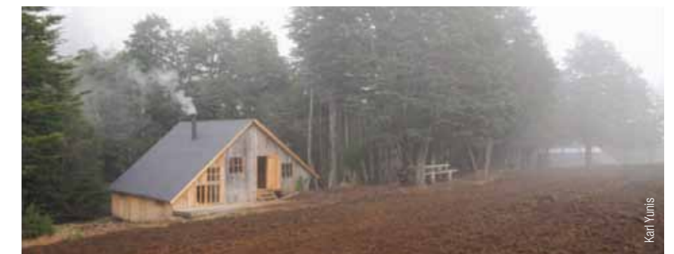
Site restoration in progress with construction of refuge for student accommodation
